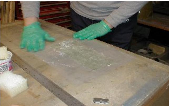
Now use your squeegee to work the resin around until all of the fiberglass cloth is completely clear and saturated with resin.
